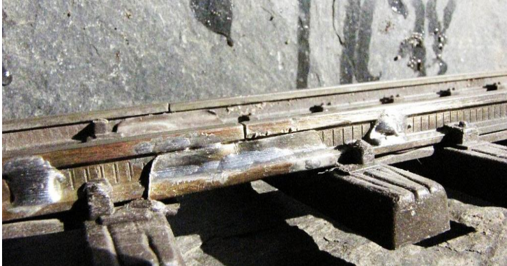
Finished Soldered Track Connections.
