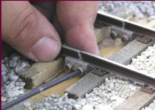
Installing Rail Clamps
